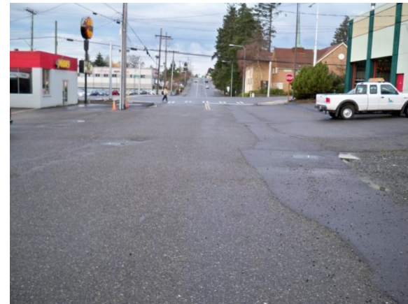
S 150 th Street 200 ft south of 1 st Ave
